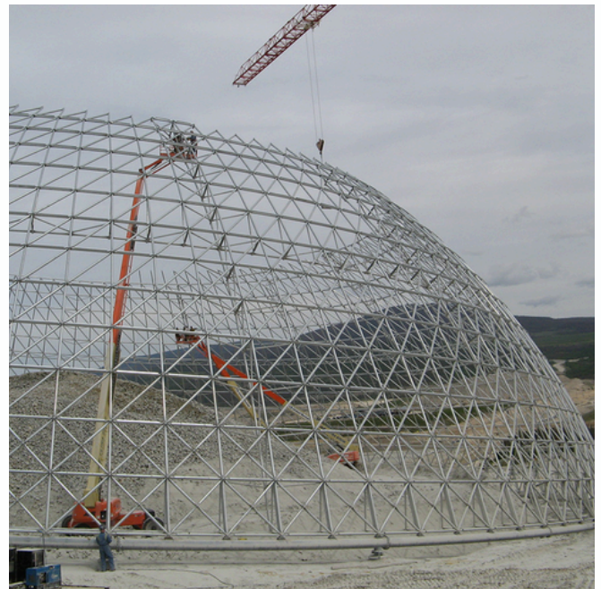
ABOVE: HVC STOCK PILE COVER AND CLADDING - GEODESIC DOMES
